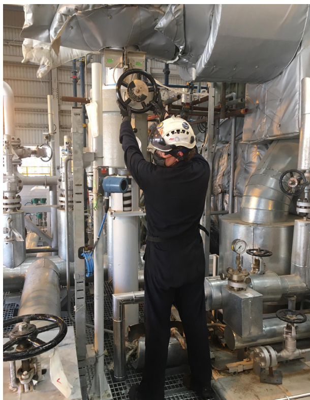
Figure 1. An AST Service Engineer operating a trip and throttle valve during a solo run.
