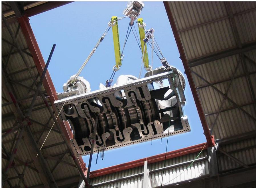
**Figure 6: Costly alternative: top half lift through compressor house roof**
